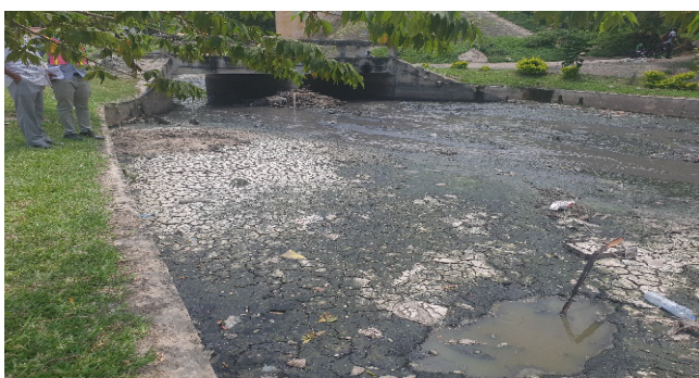
Deposition of sediments in Mpogo stormwater drain in Ilala MC
