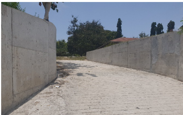
Sinza River Stormwater Drain in Kinondoni MC
